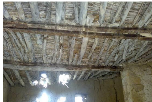
Fig. 2: Collapsed Ceiling
