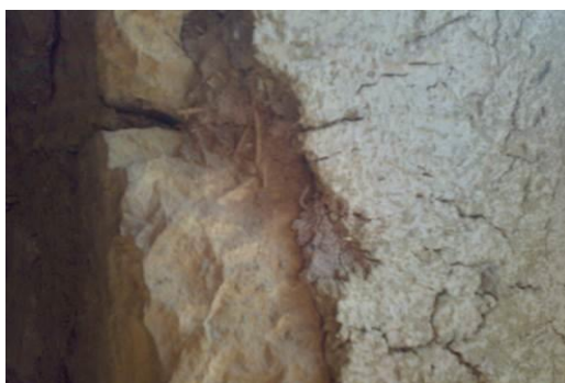
Fig. 3: Peeling plaster
