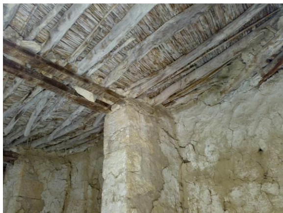
Fig. 15: The exposed wooden ceiling
