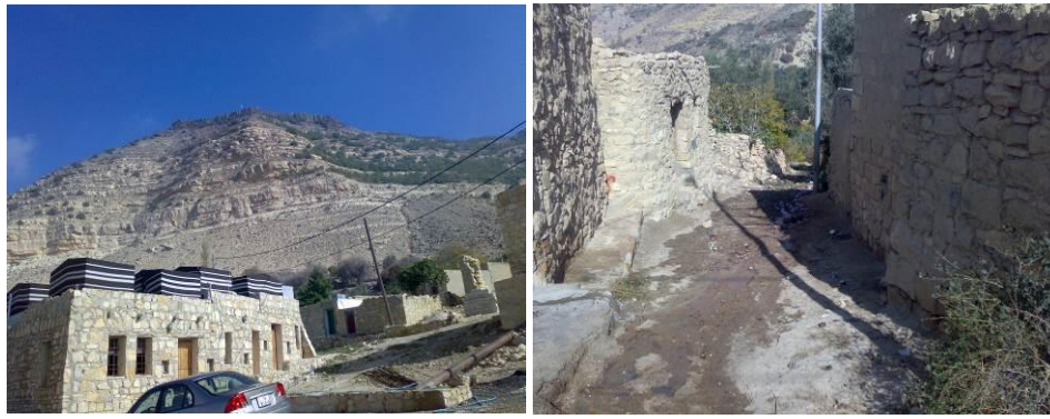
Fig. 13: Deteriorated pathways and use cars inside village paths in addition to extra roof loads.
